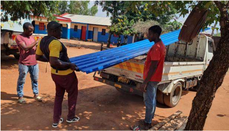
Offloading the roofing materials for the class.
